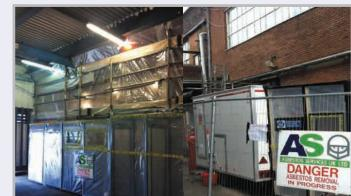
Asbestos Services UK Ltd was appointed to remove high level asbestos sprayed coatings to the structural steelwork of J block.
