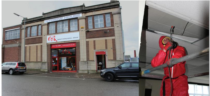
Asbestos Services were appointed by ICS Cleaning Supplies to carry out removal of high risk asbestos insulation board from internal office areas, prior to major refurbishment to the first floor level.
